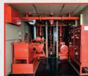
Containerised Fire Set (CFS)
